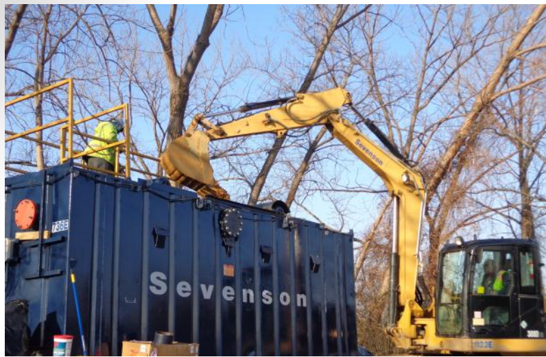
Mixing of sand and site water for slurry
