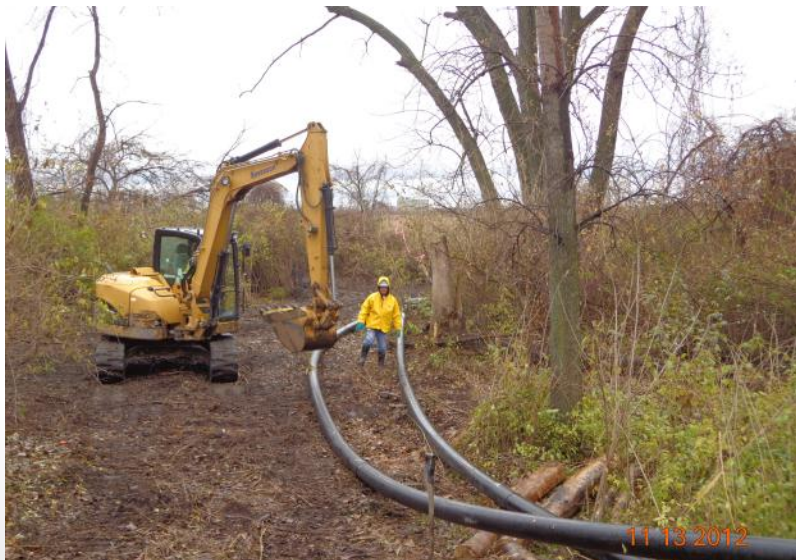
Slurry lines extended through marsh
