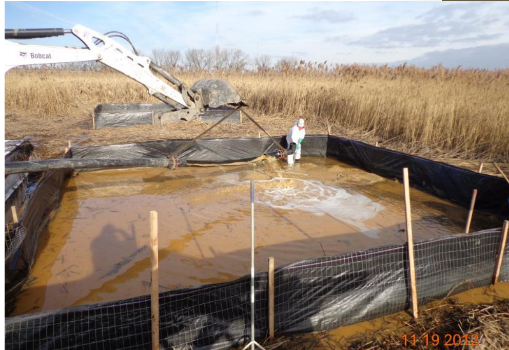
Slurry placement and grading
