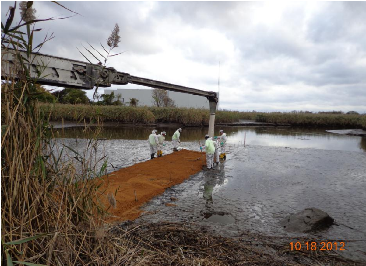
Telebelt delivery with grading to elevation
