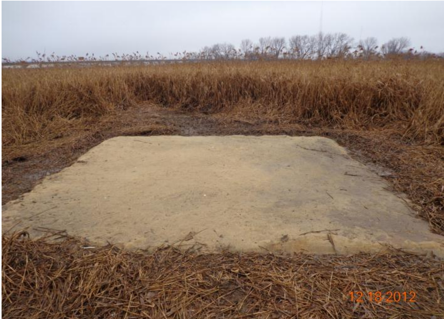
Completed test plot in marsh
