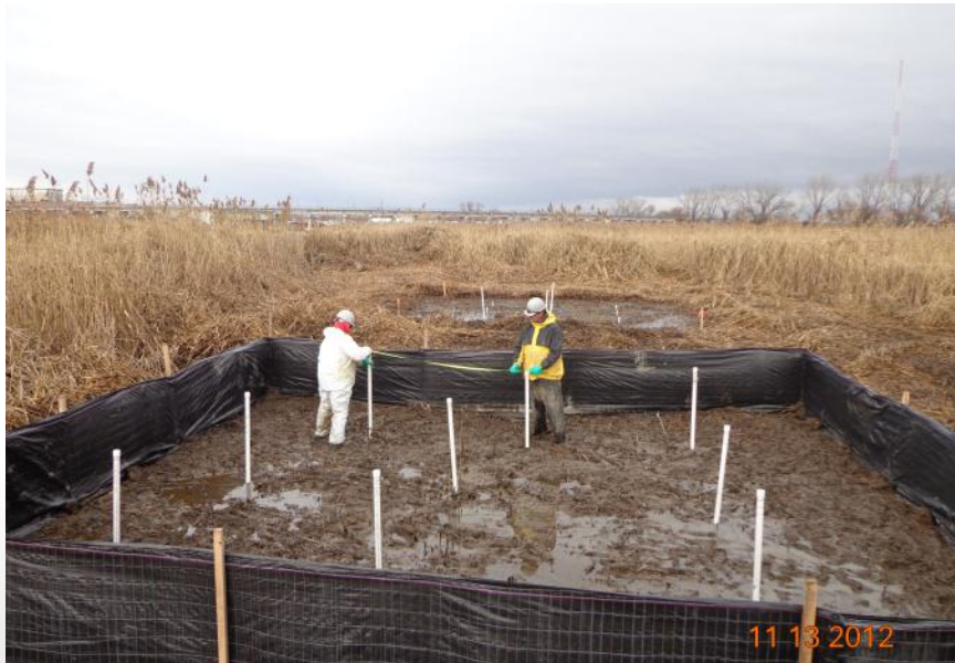
Fencing elevation stakes installed
