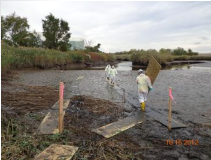
Installation of walkways
